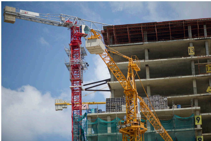
Construction work in Ashrafieh
